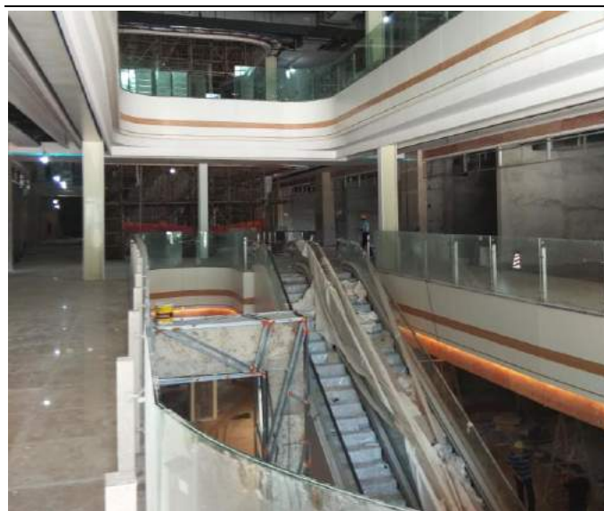
Fig 72 - Doumen Mall under construction in Sep 2018
