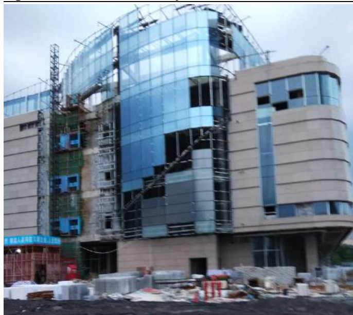
Fig 75 - Shunde Mall currently under construction
