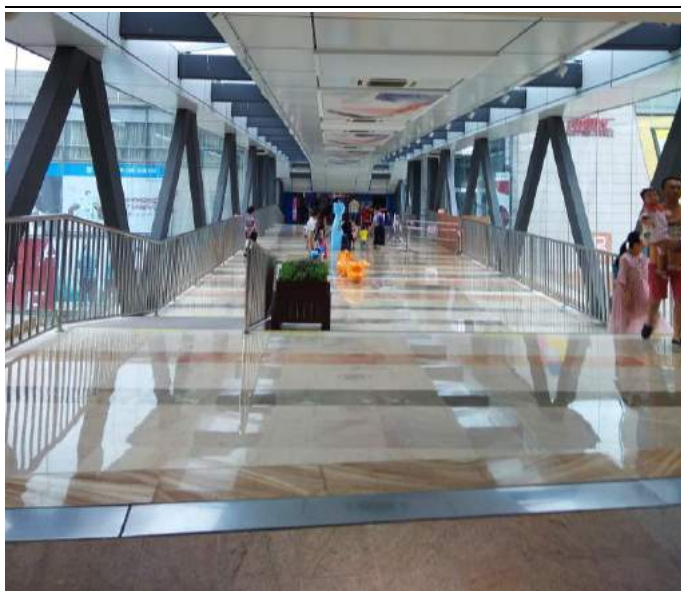
Fig 67 - Bridge that connects Shiqi A and B
